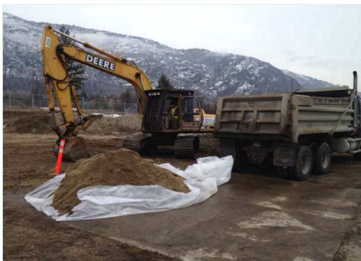
Photograph 6: Removal of hydraulic oil impacted soil. Note backfilled excavation.
