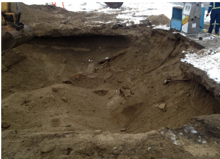
Photograph 2: Excavation upon removal of USTs and prior to pump island removal.
