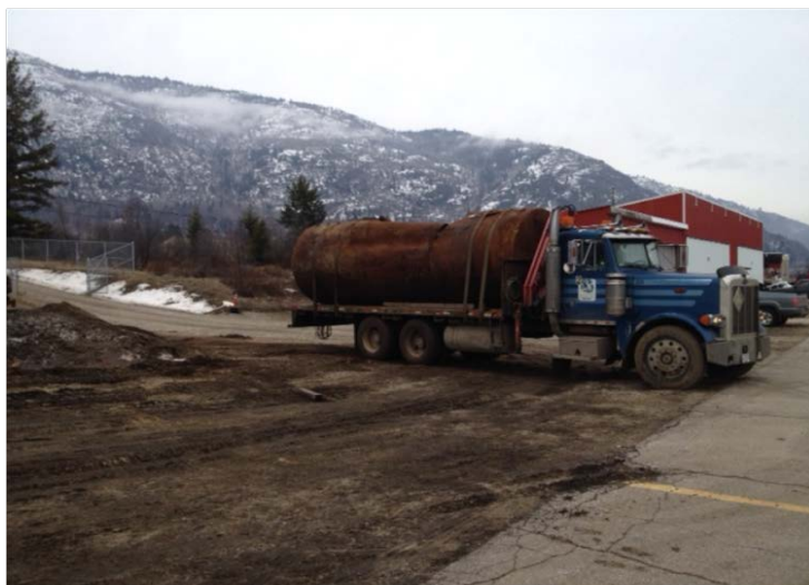
Photograph 5: Removal of UST from Site by Columbia Recycling.
