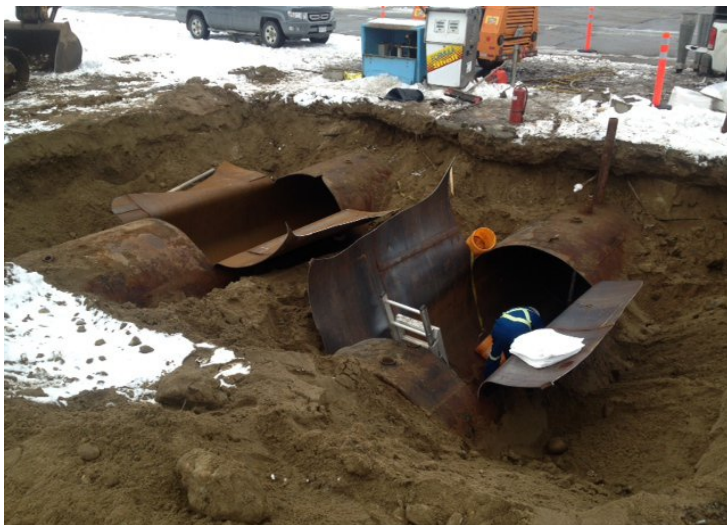
Photograph 1: USTs daylighted, purged, cut and being cleaned.
